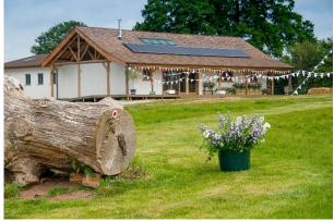
Our eco-building (above) was constructed using many natural materials that can be seen by visiting groups including hemp insulation, solid hemp walls, recycled newspaper insulation, sheep's wool insulation, welsh slate, lime plasters, clay paints and recycled aggregate paving. We also generate our own electricity using PV Panels and generate our own heat using an air source heat pump.
