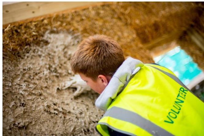
Clay being applied to the straw on our internal walls
