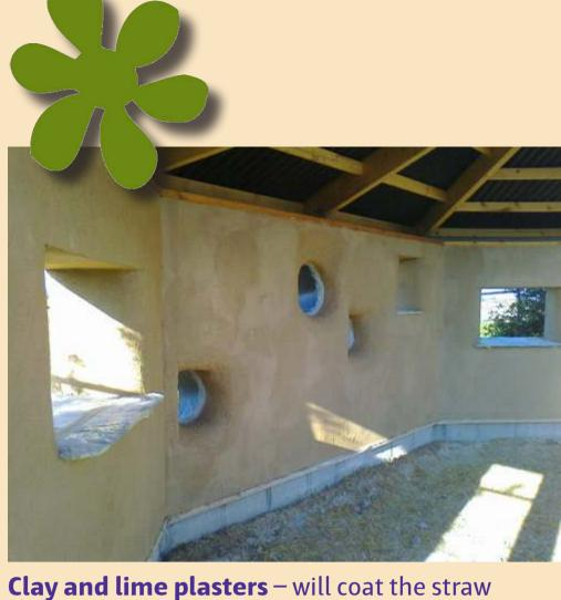
offering protection from the elements, safeguarding it from damp, providing a fireproof lining and offering a completely breathable and natural wall structure. The clay plaster will cover the inside of the walls and will all be applied by hand. It is important that there is good contact between the clay and the straw which means working it into the bale a layer at a time.
